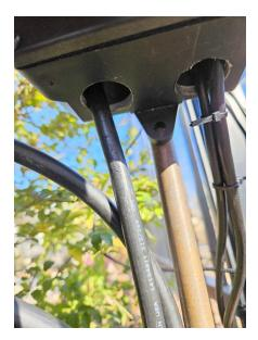
Figure 3 shows the bottom of a 4 X 4 inch NEMA box in use at N4GG to house a coax splice. Note the holes at the bottom are large enough for a PL-259 to easily pass through.
