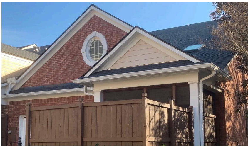
Fig 3. Gutter antenna hidden in plain sight - Note the plastic transition in the center of the pic
