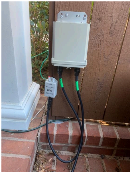
Fig 2. Remote tuner and balun installation
