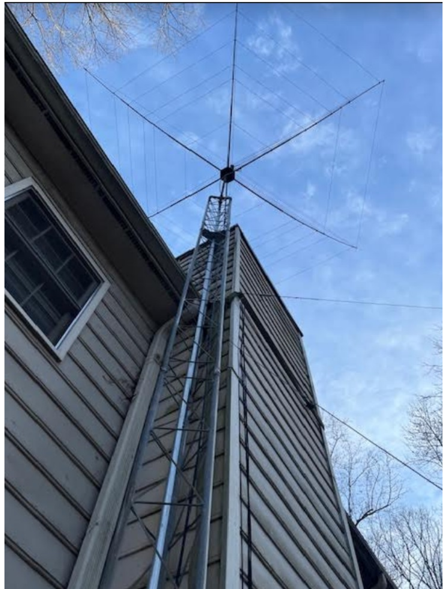
Figure #7 – The finished tower assembly in operating position
