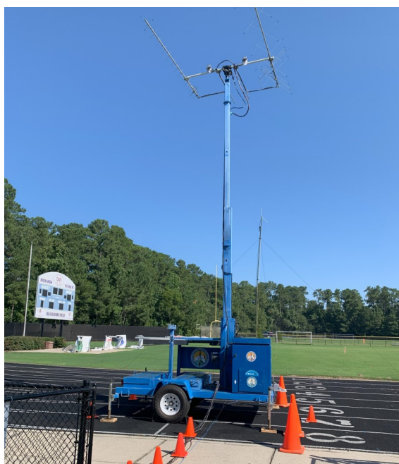
Primary antenna tower, in front & backup antenna at rear
