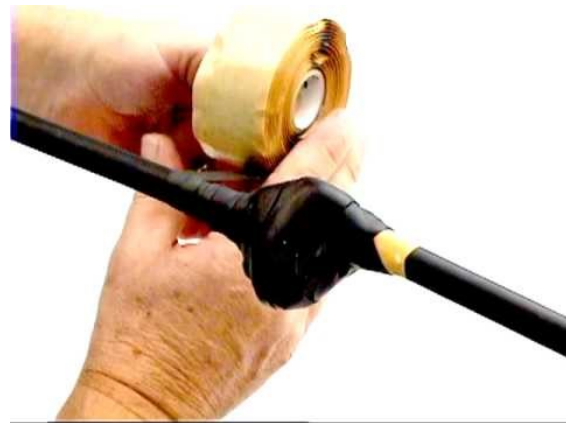
Figure 8 Scotch 2228 used to cover split bolts
