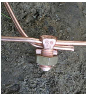
Figure 5 A split bolt tap.
